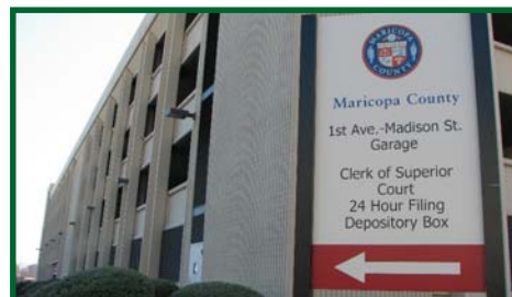
In December, the Madison St. Garage will be torn down so the new Criminal Court Tower can be constructed in its place. Clerk employees who park in this garage will begin parking in the Jackson St. Garage.
