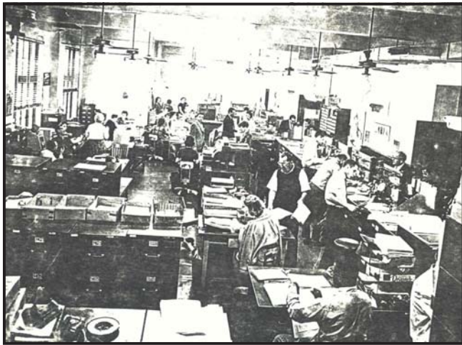
Pictured above is a scanned image of a photocopied picture of the Clerk of the Court's Office on the 2nd Floor of the Old Courthouse prior to 1965.
