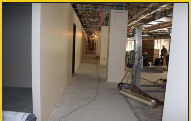
Looking east in the WCB this month.
