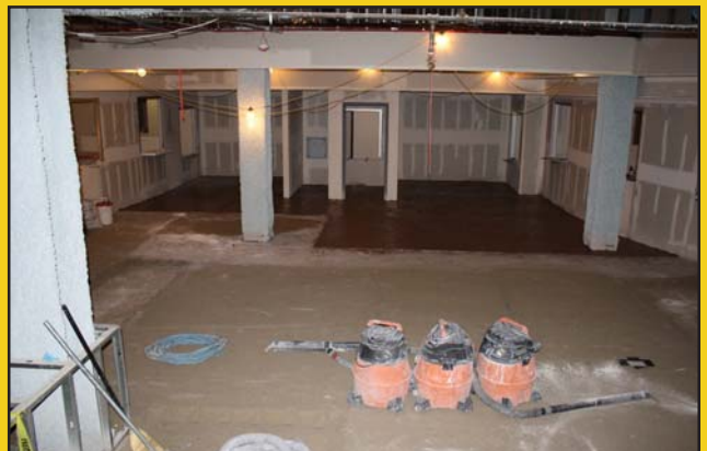
Flooring preparation for file counter lobby.
