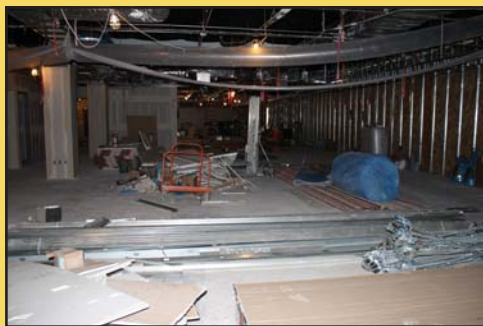
Former courtroom clerk floater pool area looking east.
