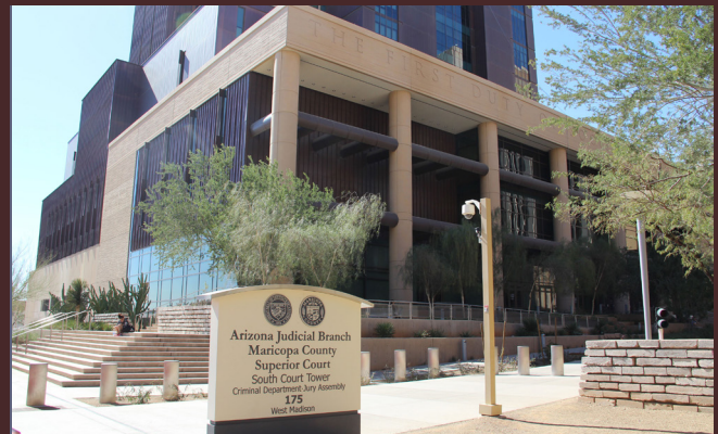
NOW - South Court Tower
